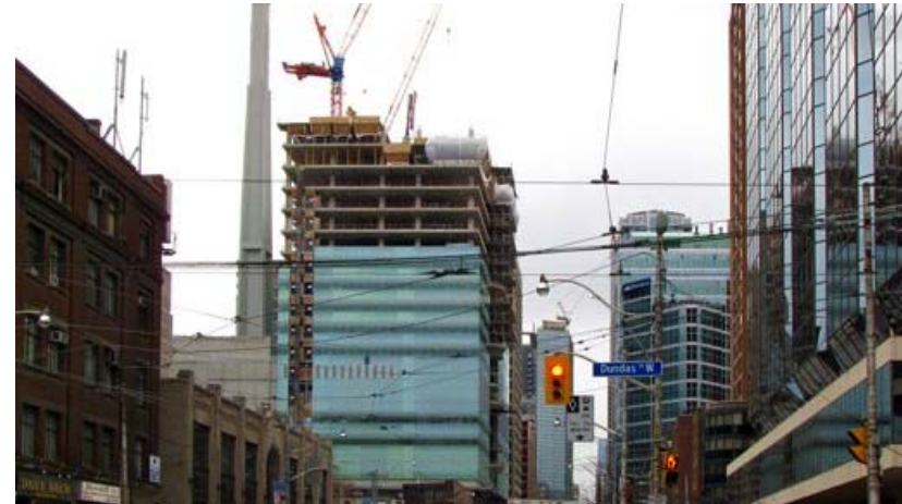
Construction progress of the SickKid Research & Learning Tower, January 2012
