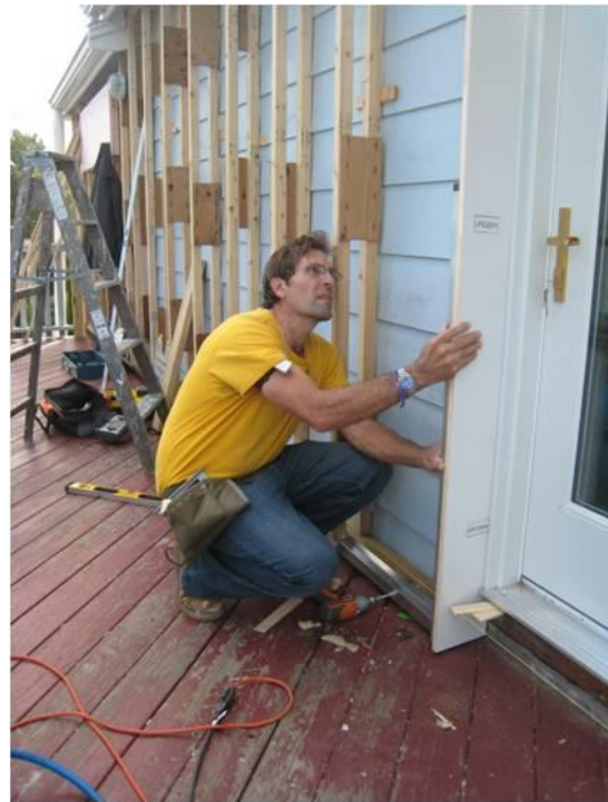
Deep retrofit with super-insulation. (source: DOER)
