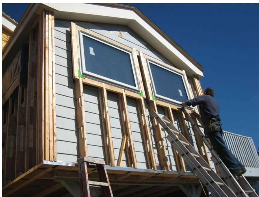
Retrofitting a house with new windows and energy efficient insulation. (source: DOER)
