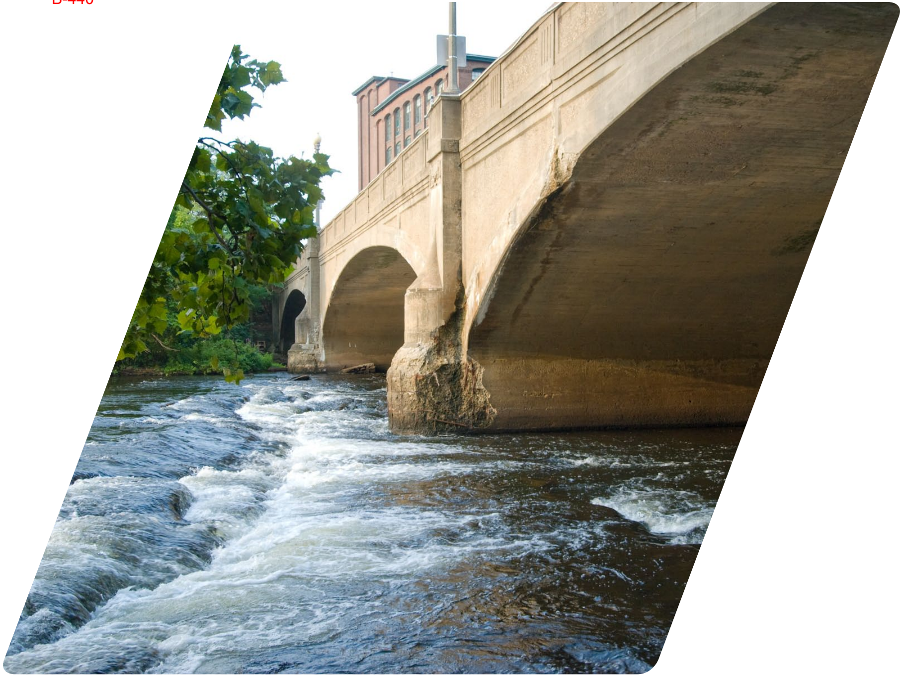
Water damaged abutments of Davitt Memorial Bridge
