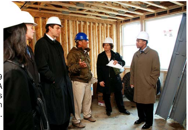
April 3, 2009 Chelsea, MA Governor Patrick’s tours rental housing construction sites.
