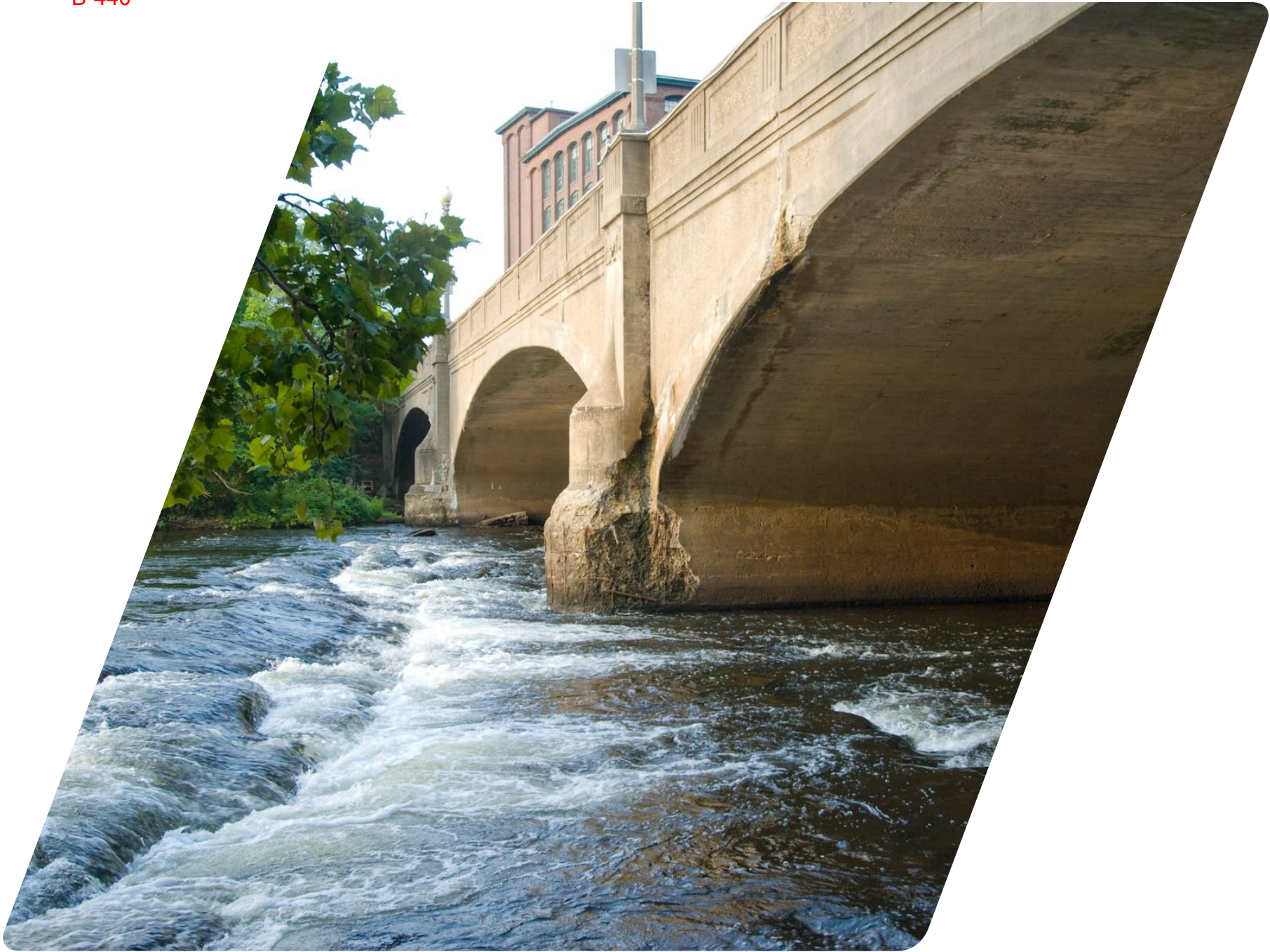
Water damaged abutments of Davitt Memorial Bridge
