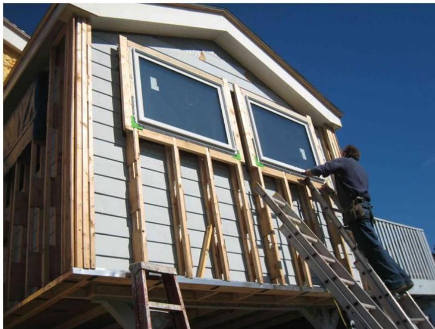
Retrofitting a house with new windows and energy efficient insulation. (source: DOER)
