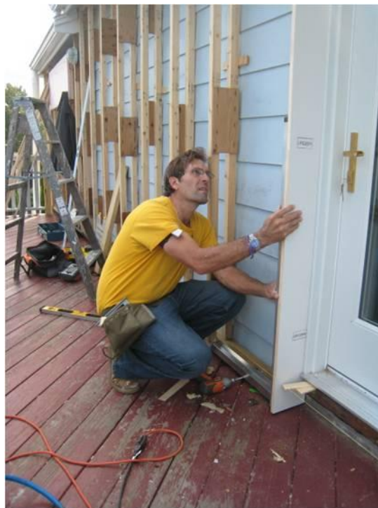
Deep retrofit with super-insulation. (source: DOER)
